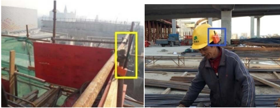
Figure 7. Tags and base stations installed on site
