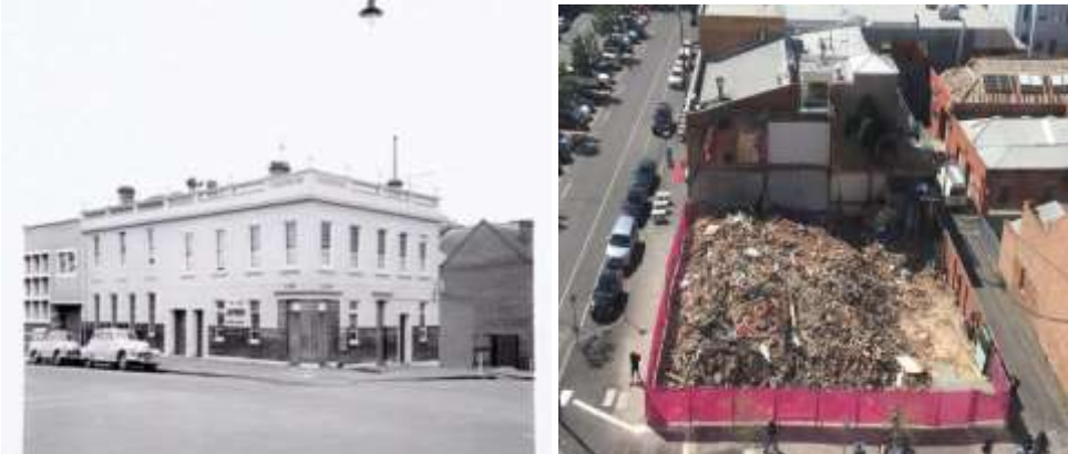
Figure 2. Before and After Demolition of Corkman Irish Pub
