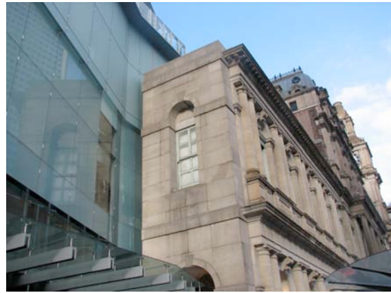
Figure 6. GPO MELBOURNE EXTERIOR (SHOWING NEW EXTENSION)
