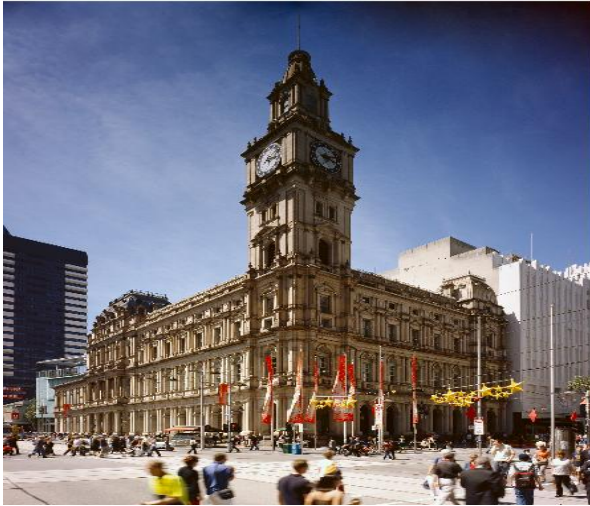
Fig. 3: GPO Building Façade
