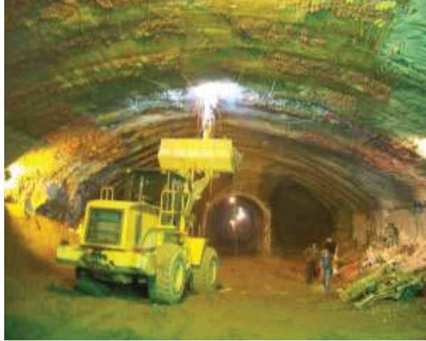
Fig 4. Construction of concrete ribs
