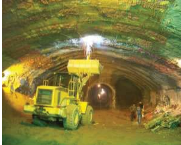
Fig 4. Construction of concrete ribs
