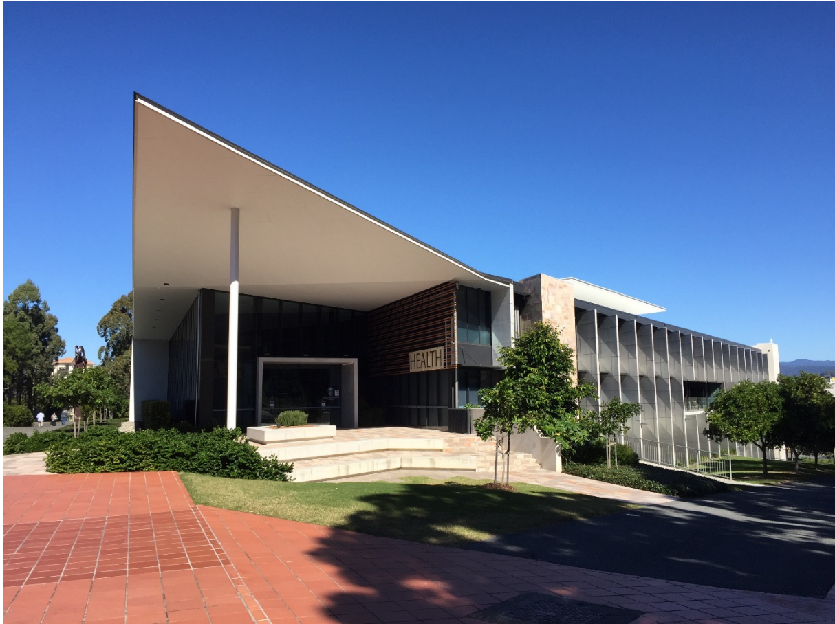
Figure 3.10. Bond University HSM Building
