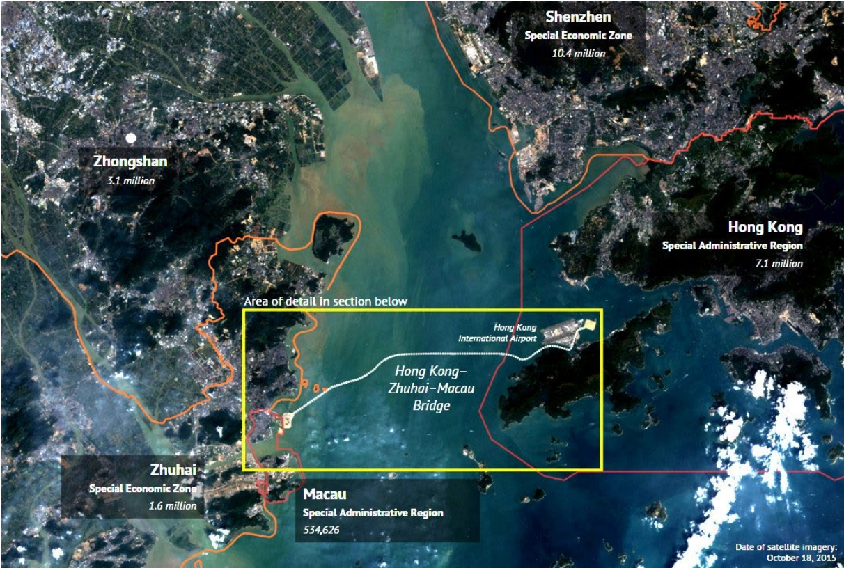
Figure 3.11. Hong Kong–Zhuhai–Macau Bridge (HZMB)
